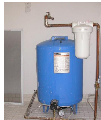
Figure 5. Example bladder pressure (blue) tank.
