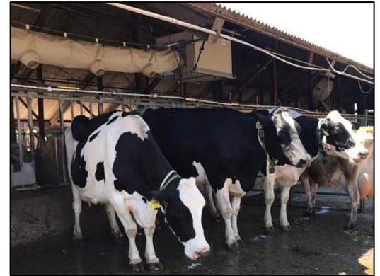
Cows line up to receive cooling from innovative direct evaporative coolers at the UC Davis dairy.
